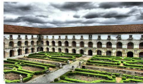
INTERIOR CLOISTER - NORTH VIEW
